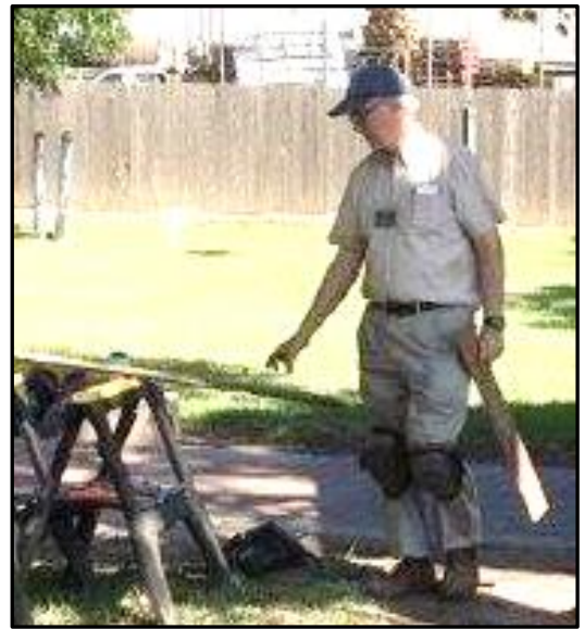
Jim Pulliam replaces wood siding on the Grist Mill/Pump House.
