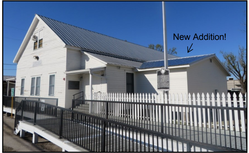
The new addition to Juergen Hall will have a small kitchen and indoor rest rooms!
